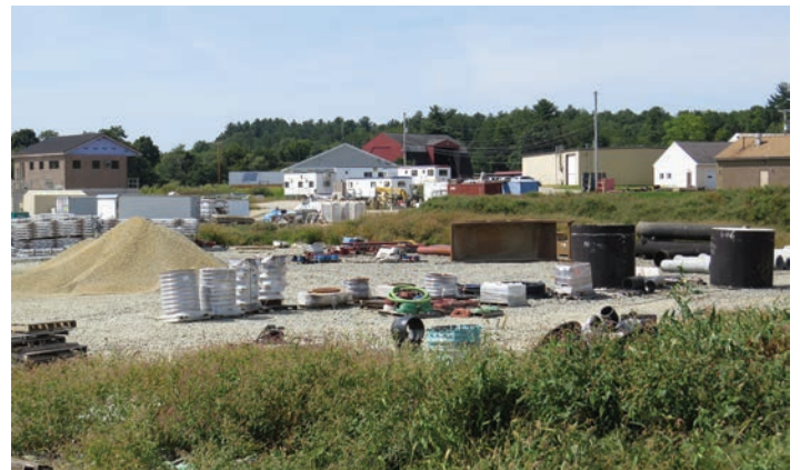
The Exeter WTP under construction. Photo by Rebecca Suomala.
